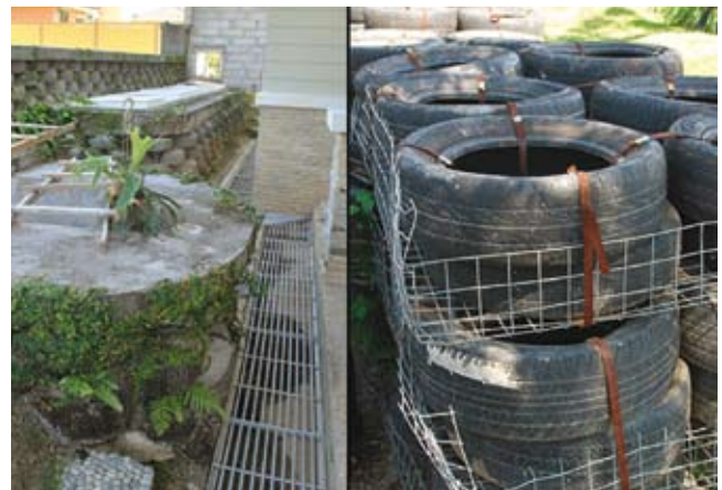
Figure 2: Tyres used as wall and tyre arrangements
