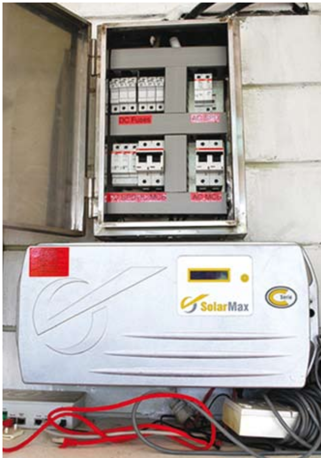
Figure 5: Solar powered distribution board and electrical DB panel to power utilities inside the bungalow
