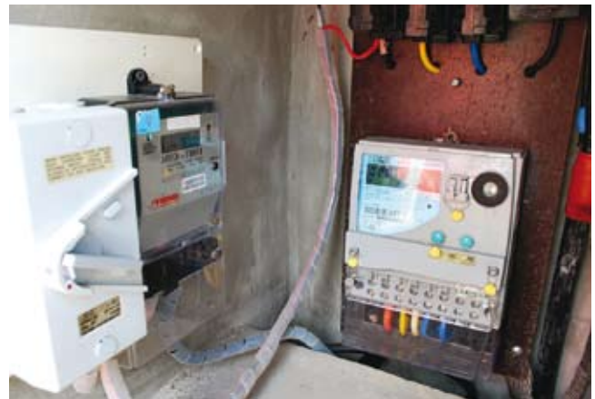
Figure 6: Solar meter: Amount sold to TNB and amount used by the bungalow
